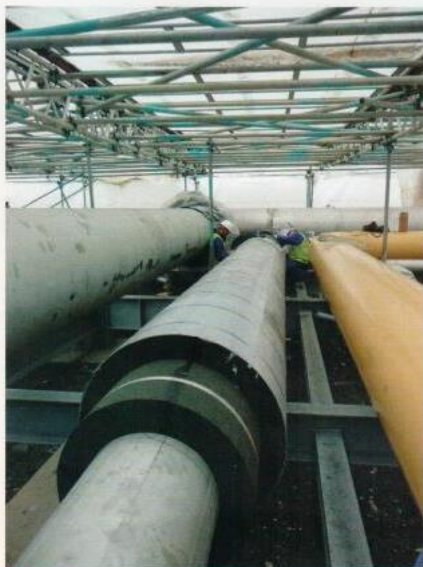
Figure 1. Pre-fabricated FOAMGLAS® insulation installed on the pipe.
