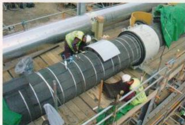
Figure 2. Installation of pre-fabricated pipe insulation system.
